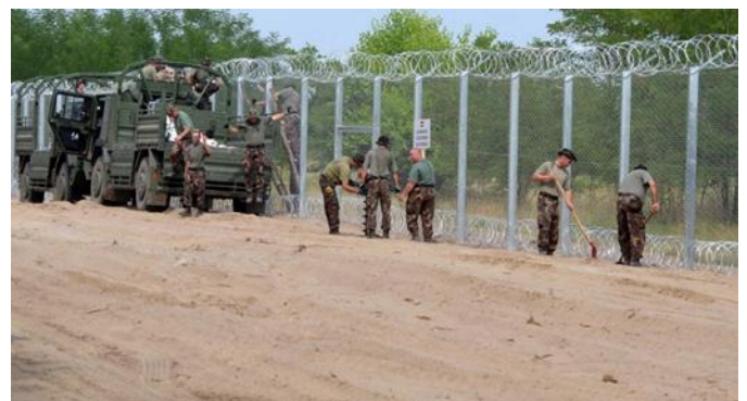
Hungarian border fences being installed
